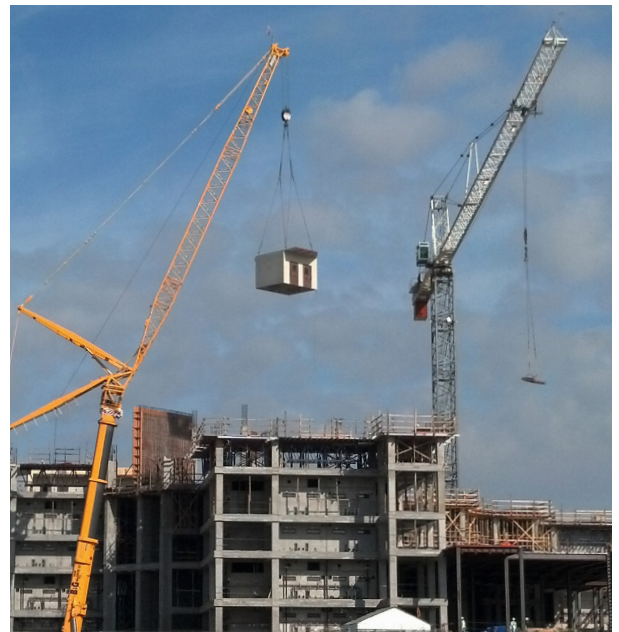
Double-cell module being erected into place
