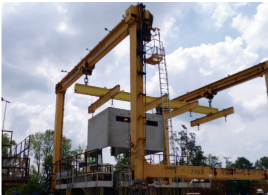
Double Cell Module being pulled from the mold
