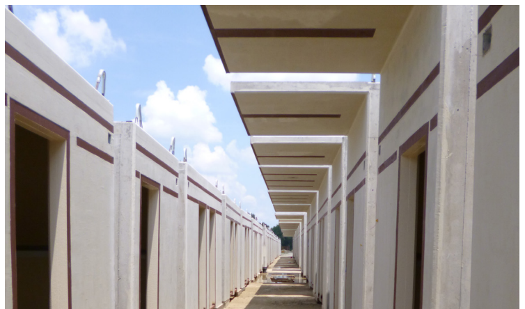
Cell Modules lined up in finish area
