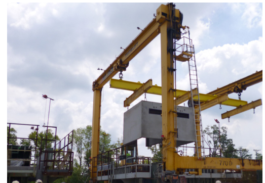
Module being pulled from the mold
