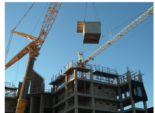
Finished module being set in place
