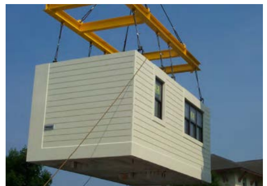
Finished module being set in place
