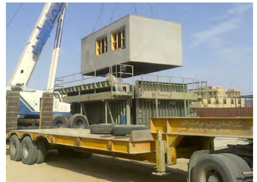
Module being pulled from the mold
